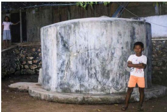
**Fig. 9 Closed rainwater storage tank**
